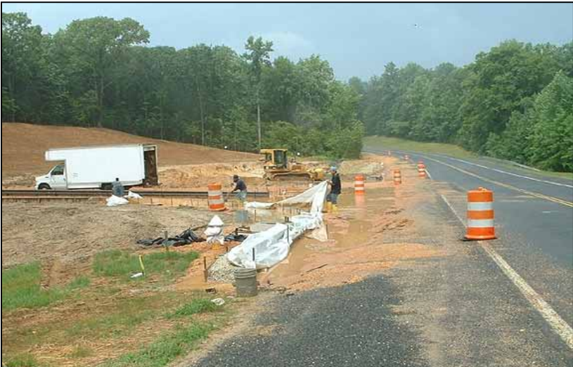
No Erosion Control at Construction Site
