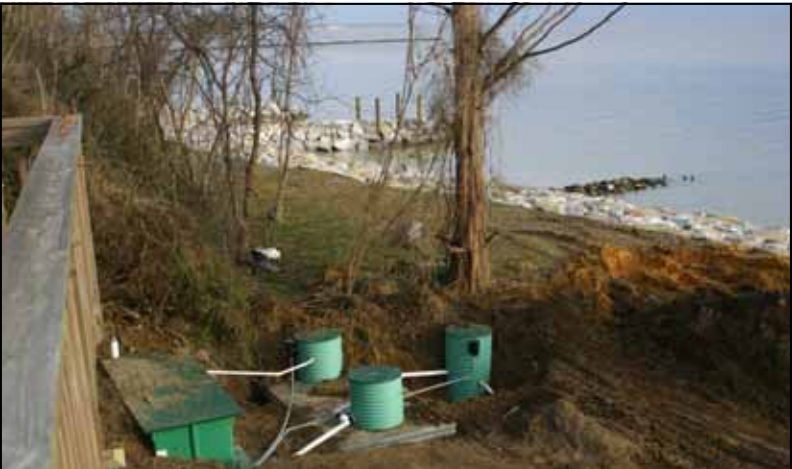
Best Available Technology (BAT) septic system during instillation
